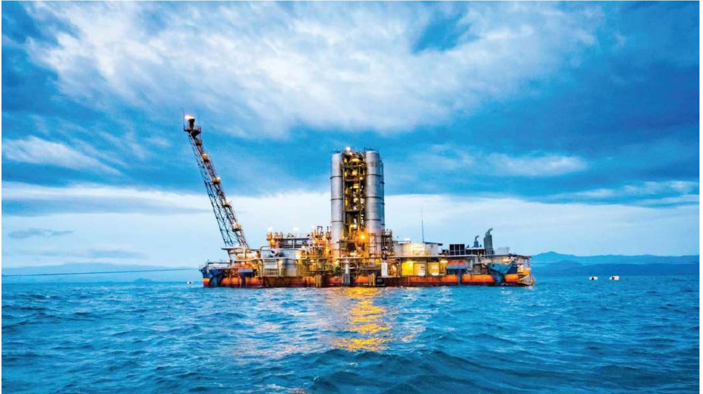
Methane Gas extraction in Rwanda
