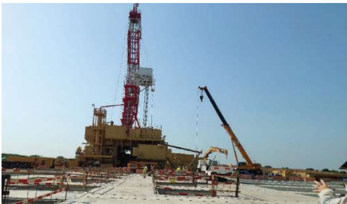
Drilling of Production wells in Tilenga Project.
