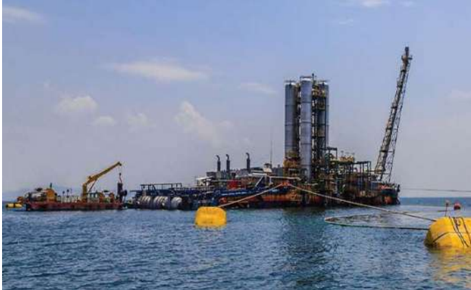
Methane Gas extraction Plant
