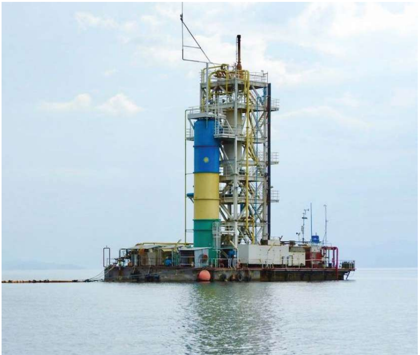
Methane extraction platform at Lake Kivu
