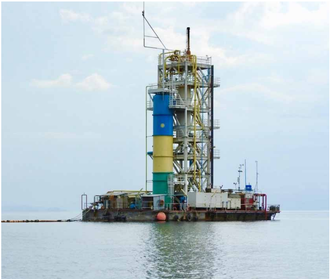
Methane extraction platform at Lake Kivu
