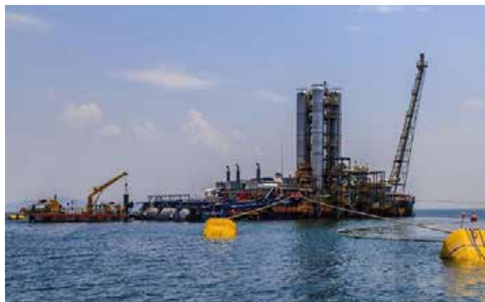
Methane Gas extraction Plant
