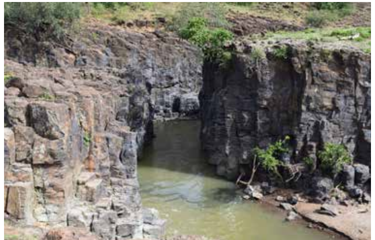
Section of the Kabarnet Trachyte at the Kerio River Bridge
