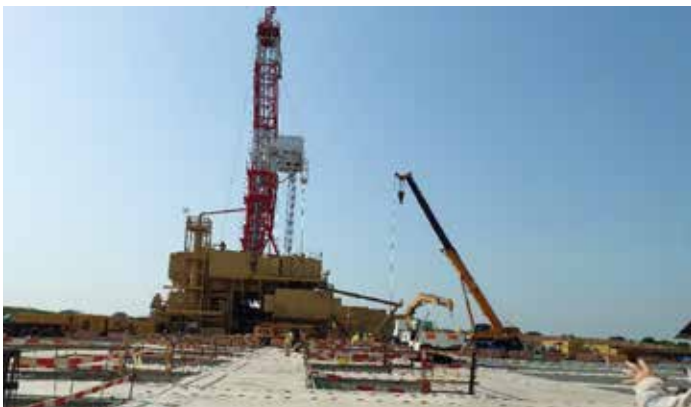
Drilling of Production wells in Tilenga Project.
