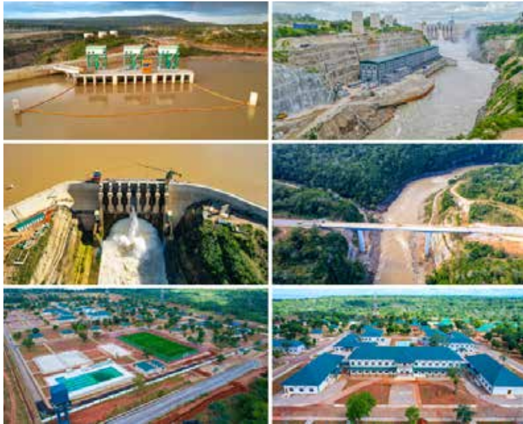
The Overview of Julius Nyerere Hydropower Project
