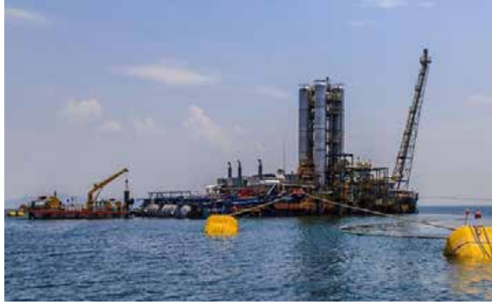
Methane Gas extraction Plant
