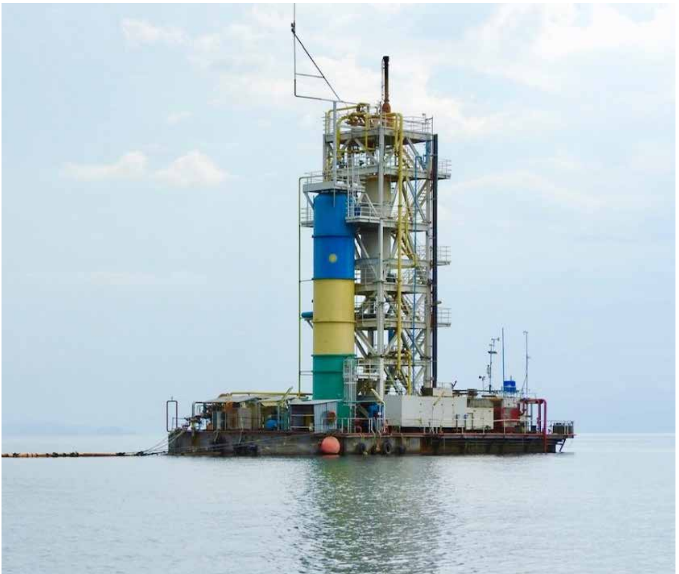
Methane extraction platform at Lake Kivu
