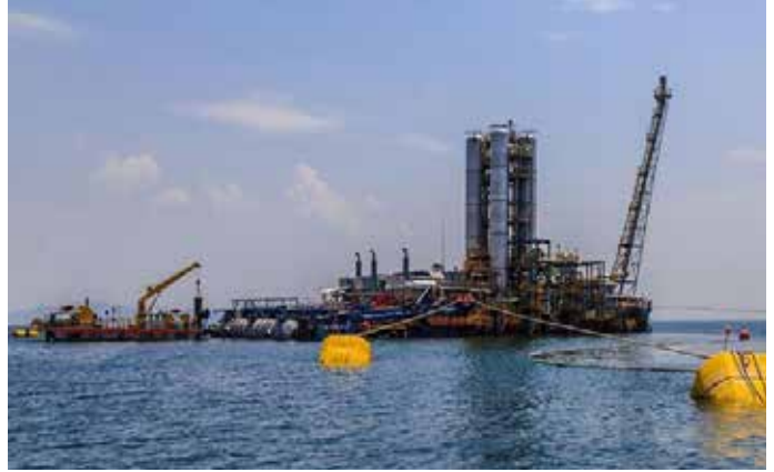
Methane Gas extraction Plant
