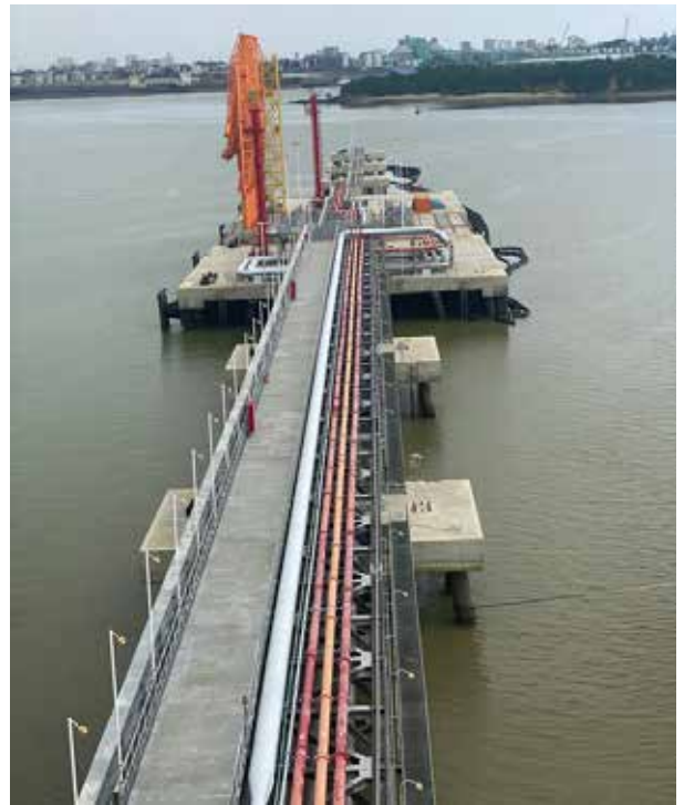
Kipevu Oil Terminal 2, Mombasa Kenya
