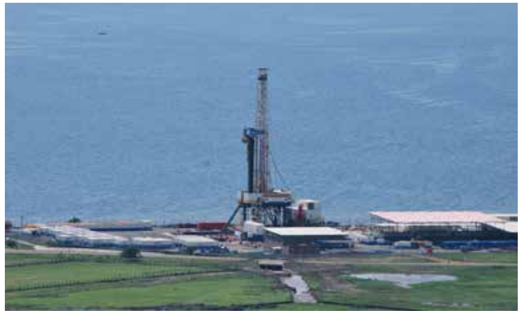
Drilling of wells at Kingfisher Development Project.
